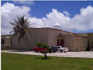
Guam Joint Region Marianas Navy Facility 2 LEO/MEOLUTs Phased Array Antenna underway; expected to be site accepted ~Fall 2026
