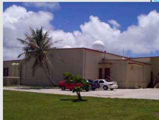
Guam Joint Region Marianas Navy Facility 2 LEO/MEOLUTs Phased Array expected operational late spring 2024
