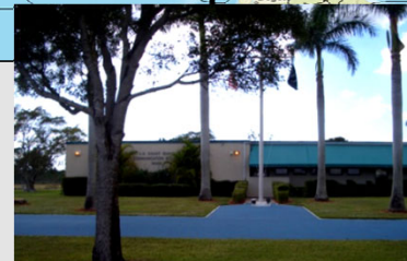
Miami USCG COMSTA 2 LEO/MEOLUTs & 6 antenna MEOLUT Refresh and Phased array funded by USAF/USCG Contracting Effort underway
