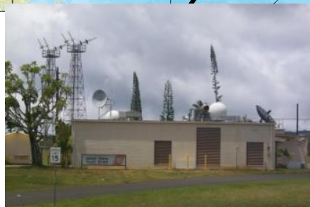
Hawaii 2 LEOLUTs replaced by 2 LEO/MEOLUTs in 2019 & 6 antenna MEOLUT
